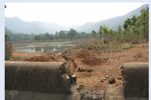
Open surplus washed away by heavy run-off from Thuajharan MIP in Chhindrapali, Gaisilat, Bargarh
