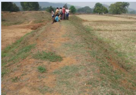
Diversion bund providing protective irrigation to fields in Chhindrapali, Gaisilat, Bargarh
